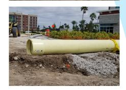
on-grade. In addition, ArrowBore offered a construction method to ensure minimal impact to traffic on the nearby seven-lane road. The replacement sanitary sewer line totaled 260 ft. of 16 in. DR 26 Certa-Lok® Yelomine® PVC pipe with restrained joint (RJ) coupled sections.
