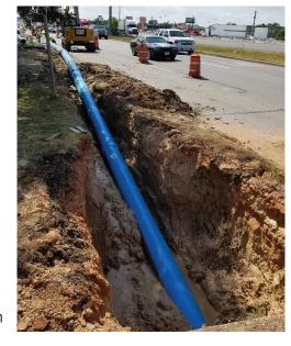
far right-hand lane, with wood blocks supporting the pipe and a small excavator lifting and moving each joint with a canvas strap. The complete pipe string was successfully pulled in under four hours. As a result, future projects to repair and rehabilitate the existing large-diameter concrete line can proceed without disruptions to water service.
