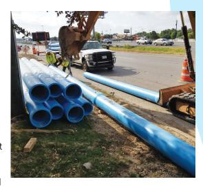
the construction of a new 12-inch distribution line that connected to the other existing distribution lines as the best solution to keep the customers in service. A major challenge identified with the installation of the new 12-inch line was a 600-foot-long, 28-foot-deep crossing of Hunting Bayou at the Centerwood Drive intersection.
