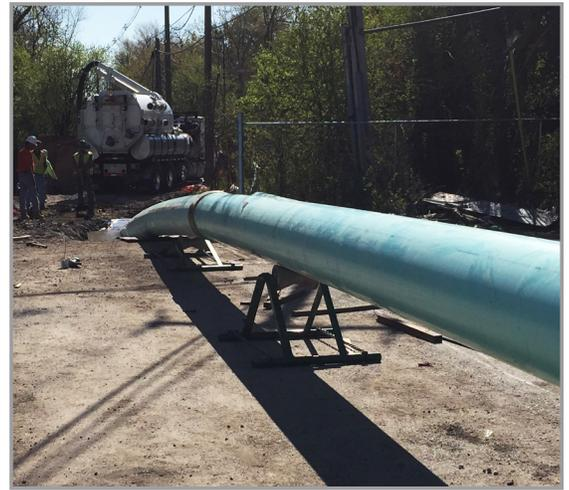
The city needed 5,000 feet of 18-inch force main; however, a good portion of this line would have to run beneath a flood plain, under levees, and cross under a creek and wetlands. For these more sensitive areas, RJN specified nearly 2,000 feet of 18-inch Certa-Lok C900 restrained-joint PVC pipe from NAPCO to be installed via horizontal directional drilling.
